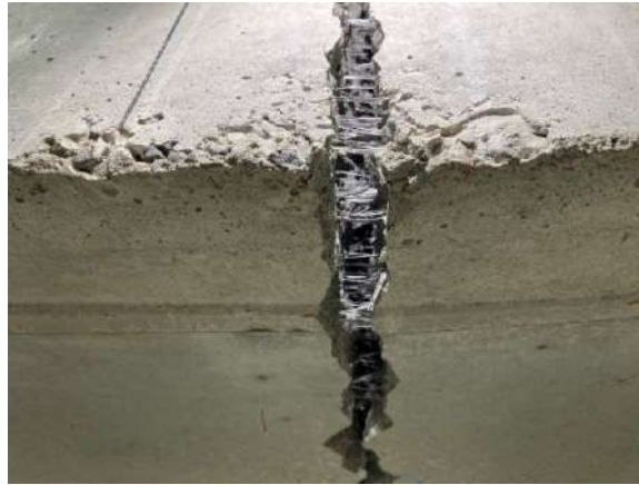
Fig. 5.32 Synthetic fibers PM maintaining the structural integrity of the tested slab 3.2
