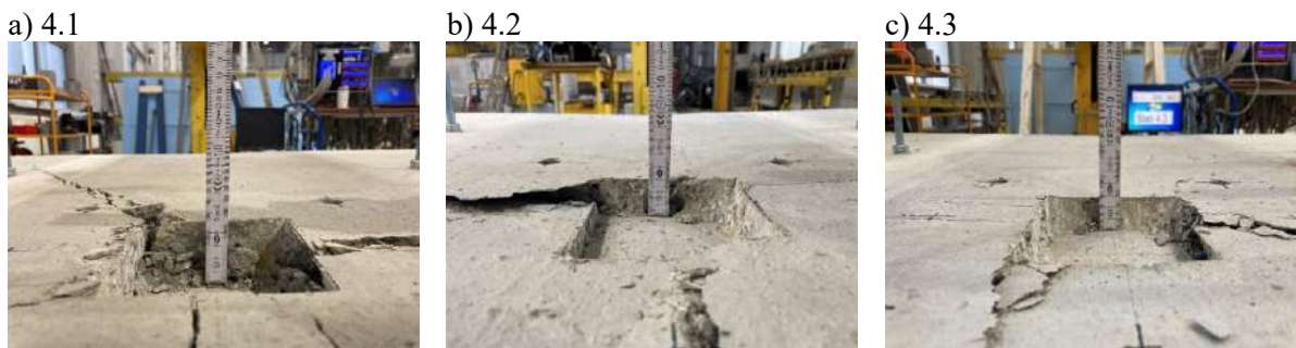
Fig. 5.43 Punching of the tested slabs of type 4 (PD_2) at the load application surface
