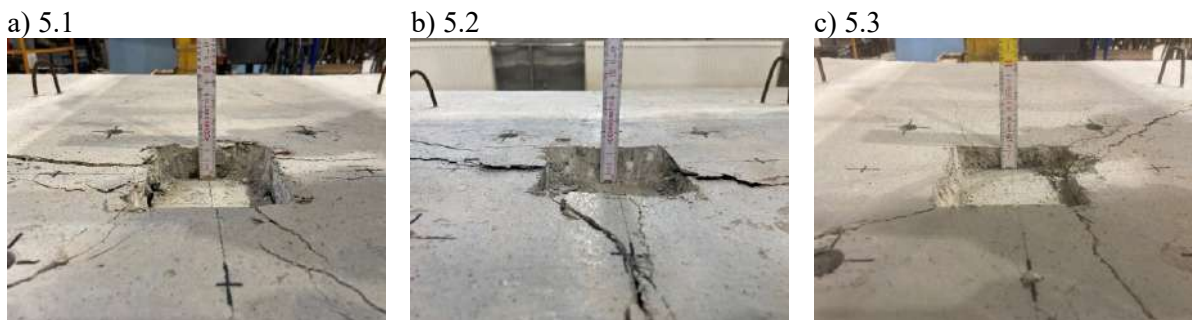
Fig. 5.50 Punching of the tested slabs of type 5 (PD_3) at the load application surface
