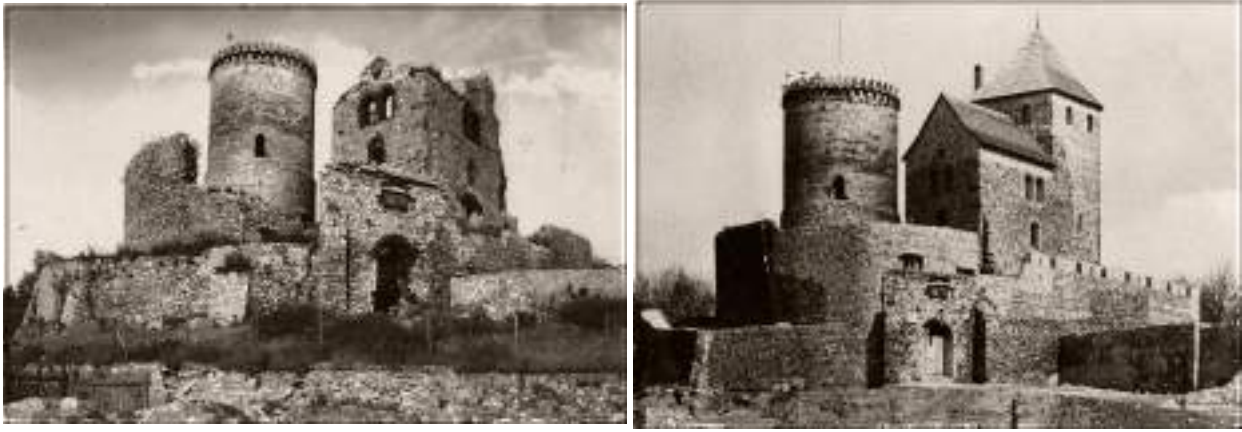
Fig. 121. Photos before and after the reconstruction of Będzin Castle according to M. Lanci's project, source: WUOZ Katowice
