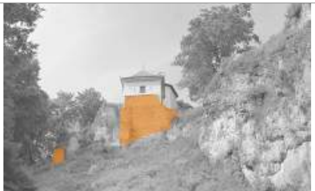
Relics of the external walls
