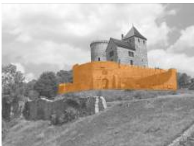
First line of defensive walls
