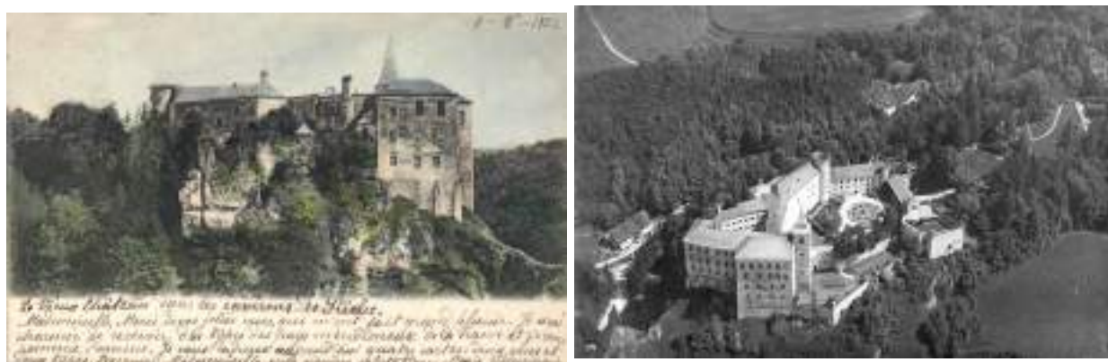
Fig. 126. The castle on a postcard from 1902 and an aerial photograph from 1930/1935, source: WUOZ Kraków
