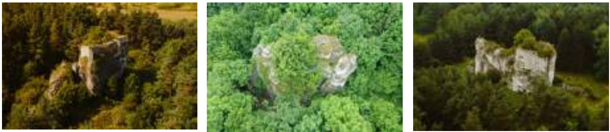
Fig. 144. Watchtower in Ryczów, Remnants of the guard tower in Suliszowice, Remnants of the guard tower in Przewodziszowice, photo by the author
