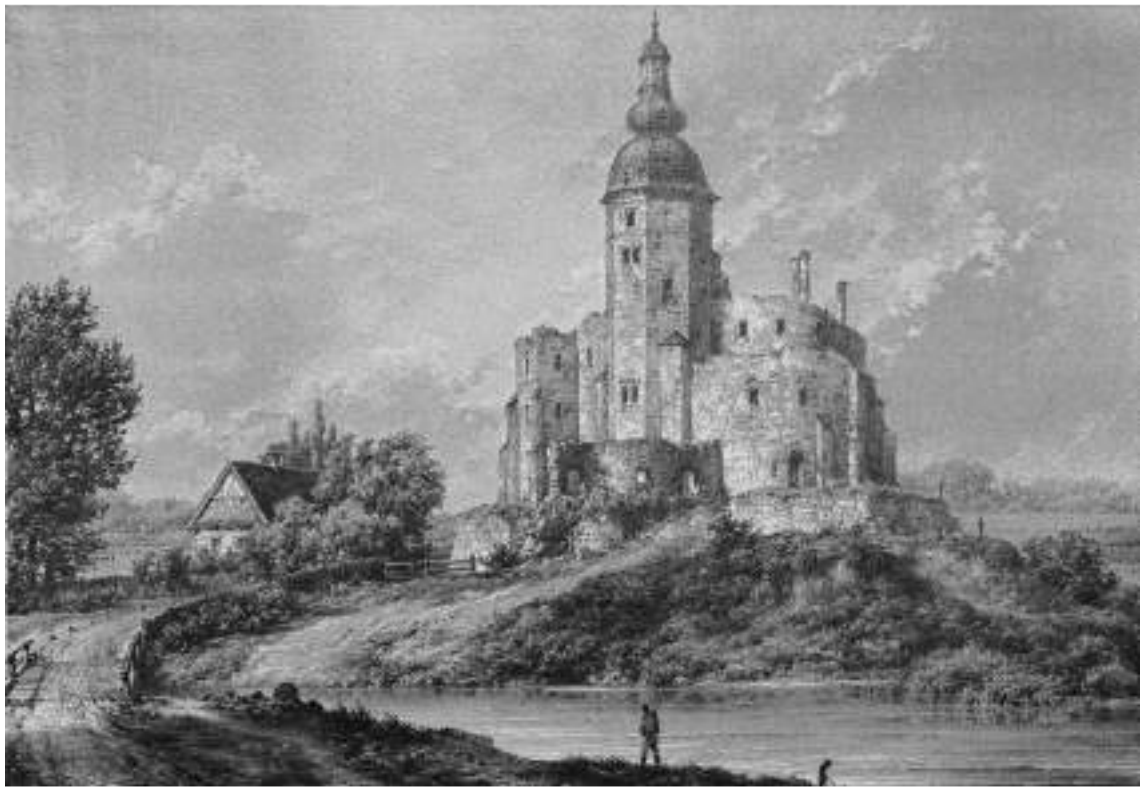
Fig. 75. View of the castle in Siewierz from 1881 on a lithograph by Napoleon Orda, source: https://medievalheritage.eu/pl/strona-glowna/zabytki/polska/siewierz-zamek/ , [access:23.05.2021]
