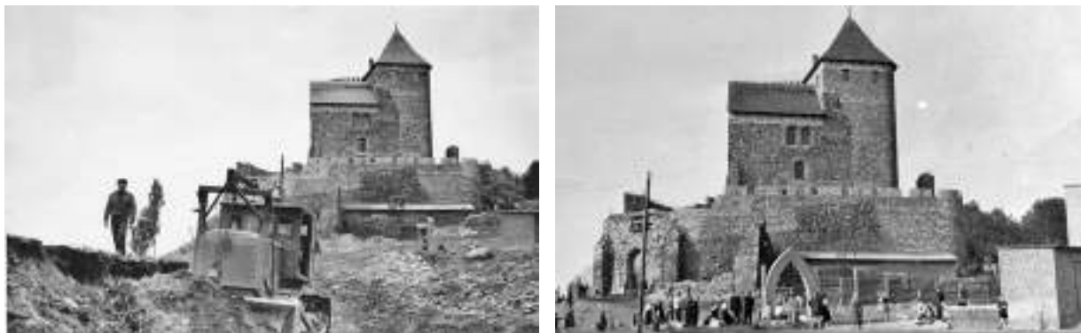
Fig. 122. Castle during reconstruction in the 1950s, source: WUOZ Katowice
