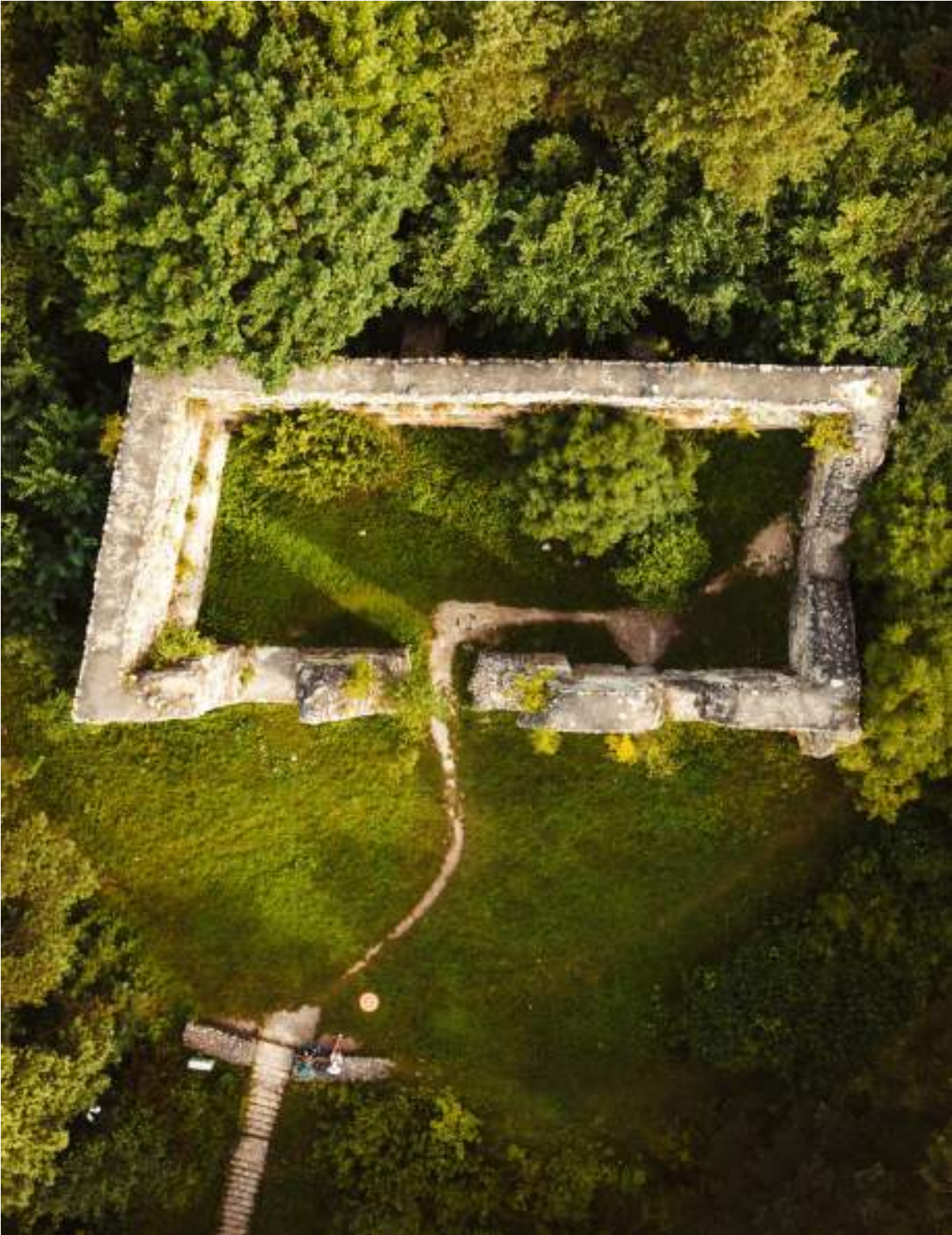
Fig. 103. External walls of the Bydlin Castle, photo by the author
