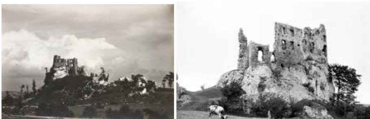
Fig. 157. Ruins of Bobolice Castle in 1932-1939, source: National Digital Library Polona, Ruins of Bobolice Castle in 1954, source: https://fotopolska.eu/Bobolice/b283,Zamek_w_Bobolicach.html?f=1995239-foto , [access: 23.05.2022]
