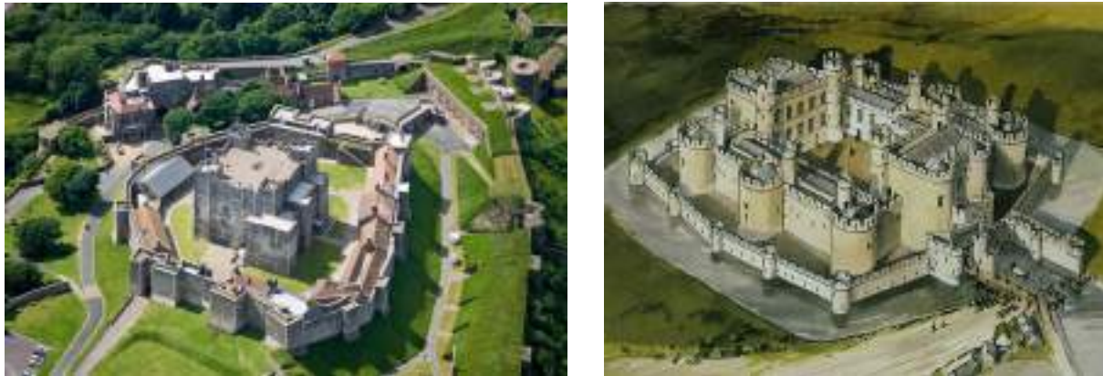
Fig. 21. Dover Castle, Beaumaris Castle, Beaumaris Isle of Anglesey, Wales. source: https://www.historyextra.com/ , https://www.castlesandmanorhouses.com/photos-wales.htm , [access: 17.03.2021]
