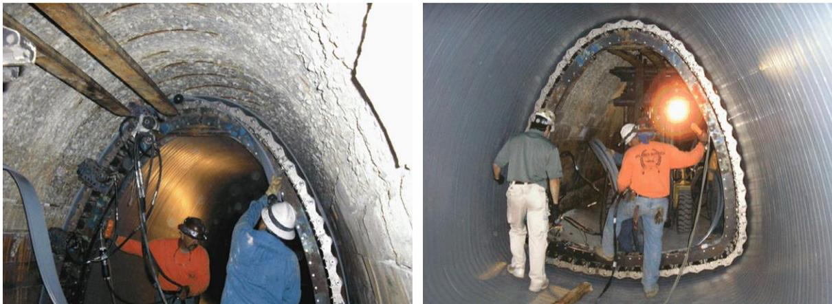
Fig.2.4.2: Sewage pipeline during and after rehabilitation [230].
