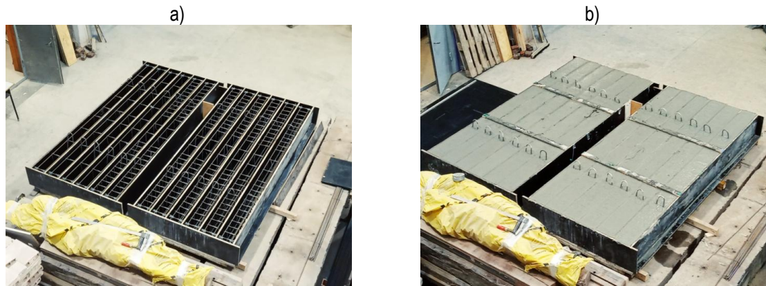
Fig. 4.6 a) Beams before pouring concrete b) Beams after pouring concrete
