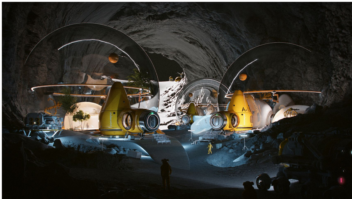
Fig. 28. Lunae Abyssi habitat located within a lunar lava tube. Visualisation showing double inflatable structures and the rigid core of the modules (courtesy of the Lunae Abyssi team).
